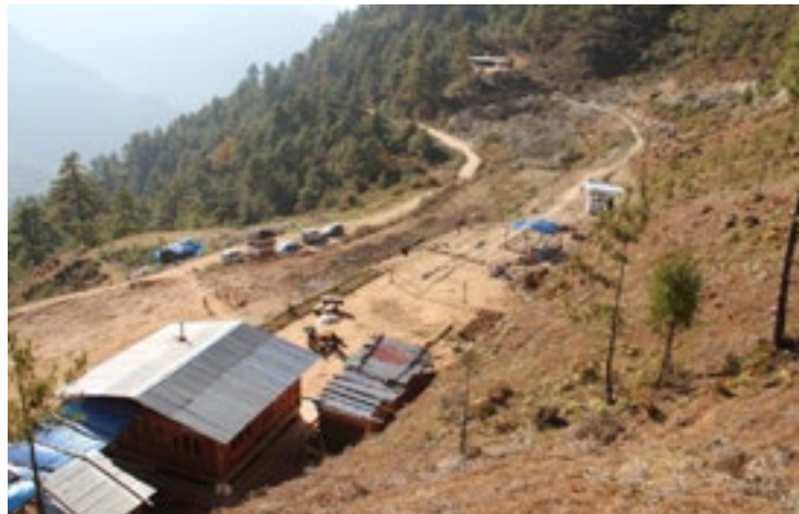
Aerial View of the CBCC
