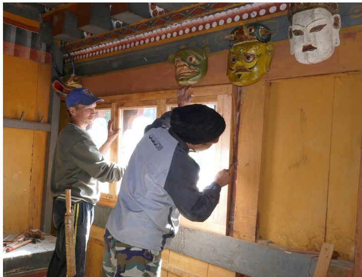
Fixing a window frame
