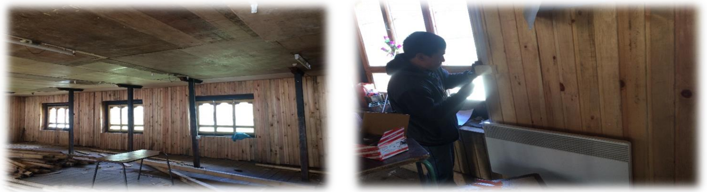
Wooden paneling and electrical retrofitting of classrooms in Mera Primary School
